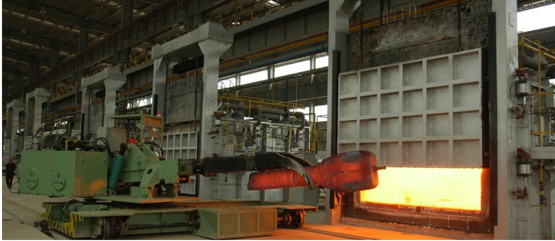
Heating furnace (table type)
